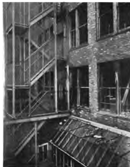
Fig. 2. Fire Escape on Plant in Newark, N.J., after Fire.*
